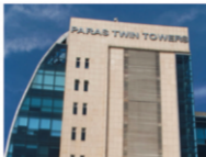
PARAS TWIN TOWERS
